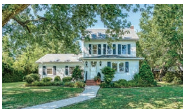
CHINCOTEAGUE 56241: Charming 2BR/3BA colonial on large commercially zoned lot. Super-sized deck overlooking the manicured grounds. Full house & garage Generac generator; many updated appliances. $499,000
