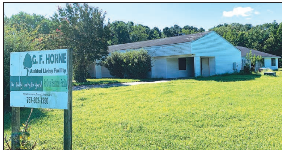
The former G.F. Horne assisted living facility in Onancock stand empty and in need of repair. The Eastern Shore Coalition Against Domestic Violence recently purchased the property to house client services and administrative offices. Photo by Connie Morrison.
