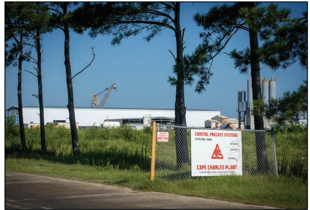
A large, new building to enclose some operations close to the Cape Charles Town Harbor stretches behind the sign greeting visitors to the Coastal Precast Systems plant. Photo by Jim Ritch.
