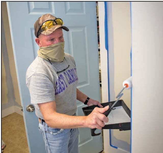
Tom Arnold, of Franktown, rolls paint on a wall.
