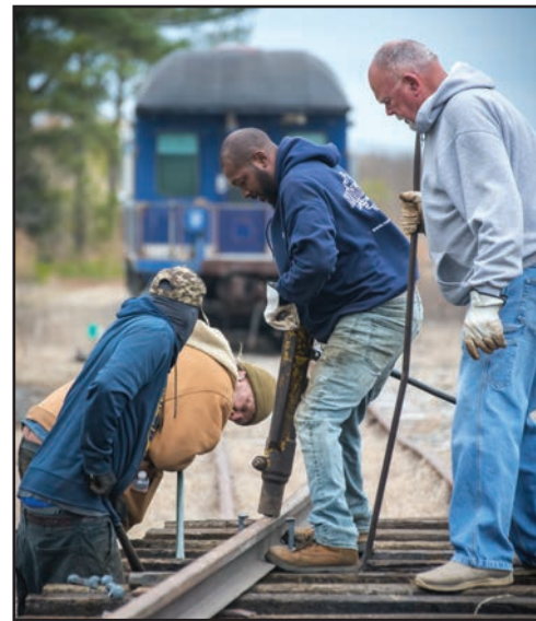
Above left: Garnesey Sanders, of Cape Charles, lifts a 90-pound jack hammer into position before driving a railroad spike into place. Holding the track and ties in position are, from left, Michael Sample, of Treherneville; John Paffrath; Sanders; and Chuck Rickman, of Roanoke, Va.
