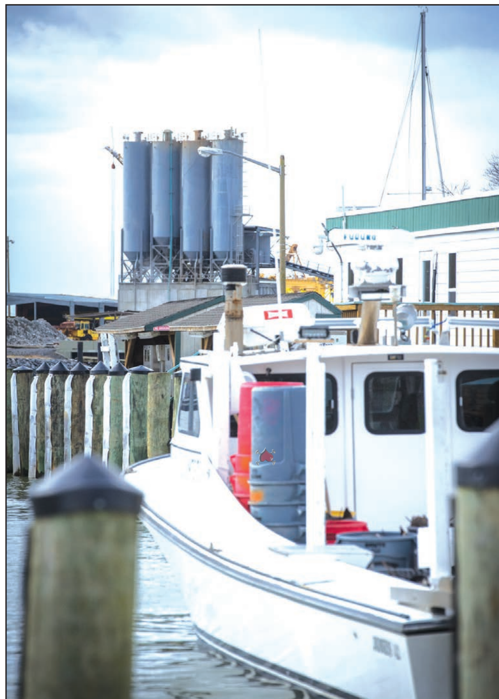
A workboat is docked at the Cape Charles harbor. The Coastal Precast Systems plant is in the background. Photo by Jim Ritch.
