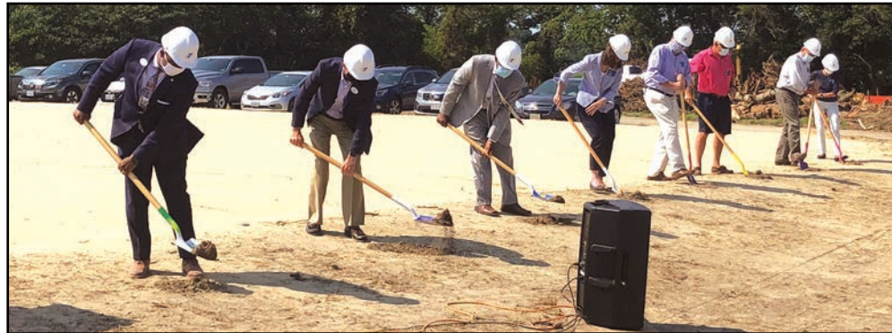
Dignitaries put shovels to soil at the Northampton YMCA groundbreaking. Submitted photo.
