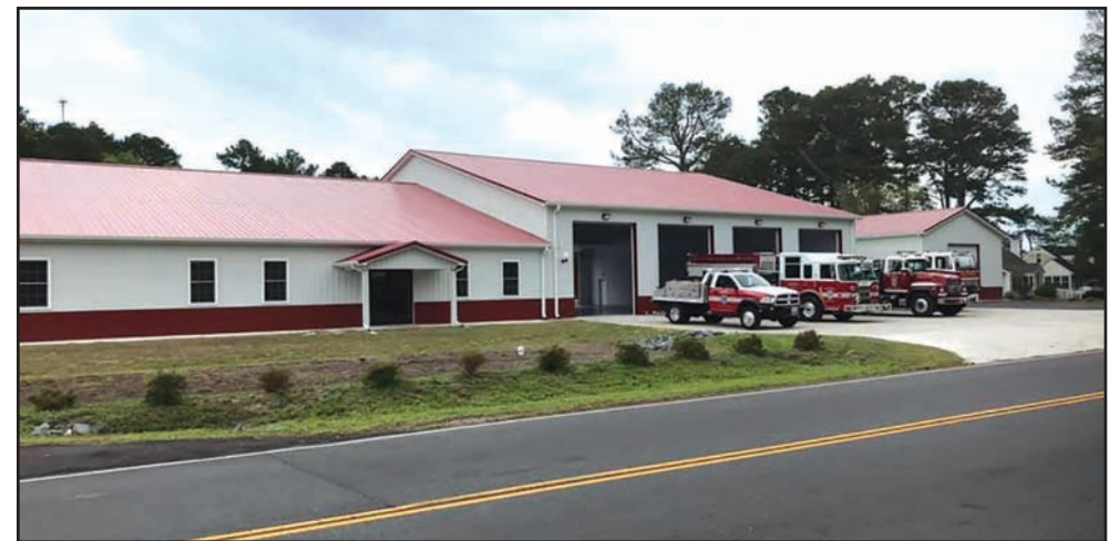
Equipment is lined up at the new Tasley Volunteer Fire Company fire house on Saturday, July 11. Photo courtesy of Tasley VFC.
