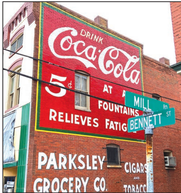
A recently renovated vintage advertisement on the side of a building is part of Parksley's small town charm. Photo by Carol Vaughn.
