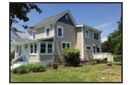
RENO'd CLASSIC 2-STORY wood floors, baths on 2 flrs. huge scr.porch/workshop $238,000
