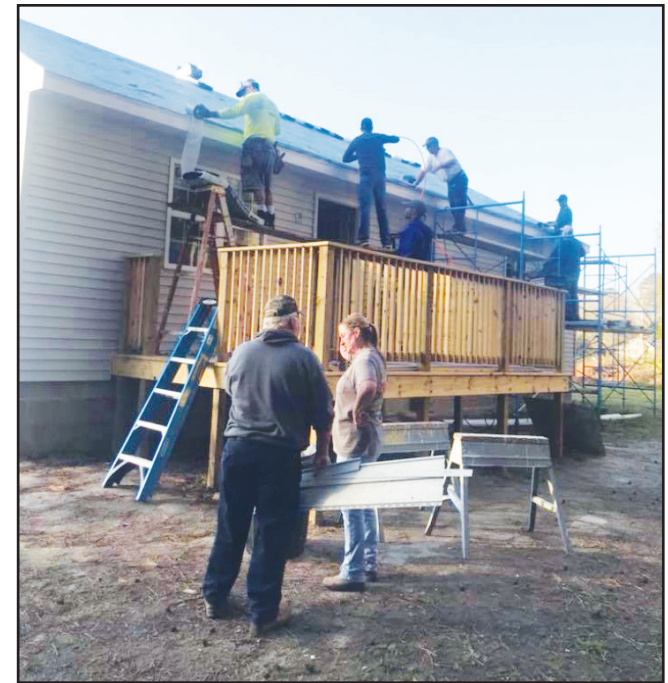
Submitted Photo Volunteers at work roofing Habitat for Humanity House No. 46.
