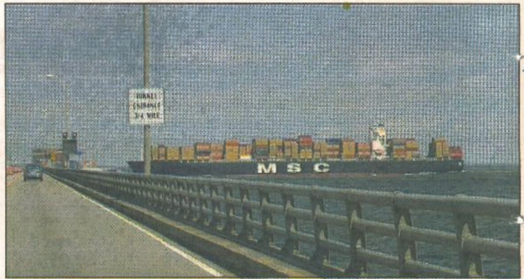
On a recent day, it appeared this loaded barge was headed for a collision with the bridge-tunnel.
