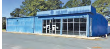
8,300 Highway-front Showroom/Retail. Former auto parts store. Belle Haven
