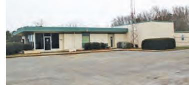
4,500 sf. office/small manufacturing fully-leased property in Onancock
