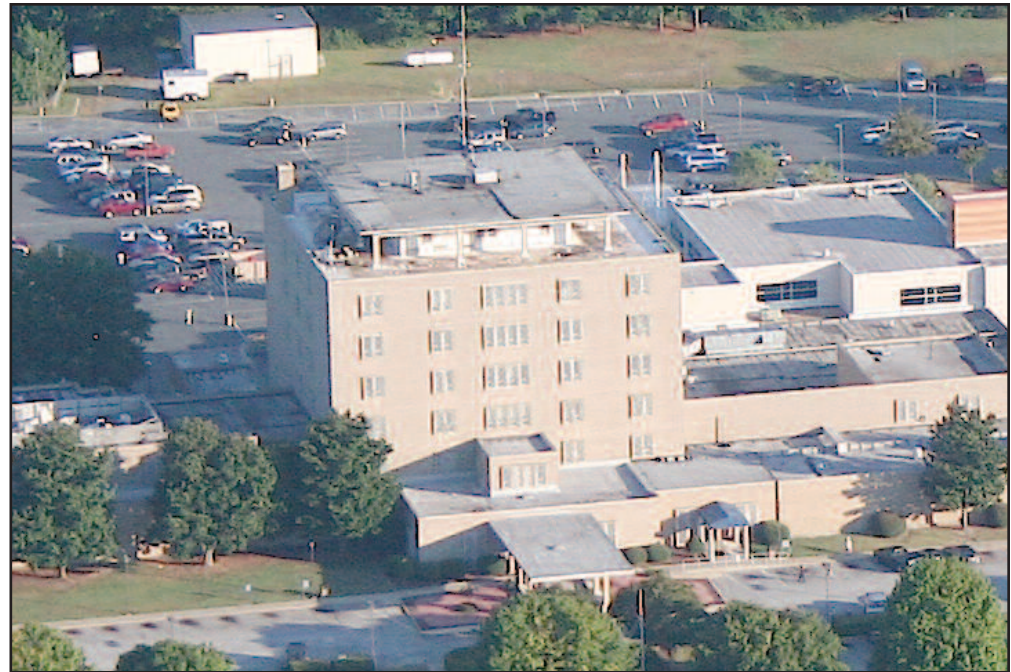
Rising above the Nassawadox landscape, Shore Memorial Hospital finds itself looking for a new owner.
