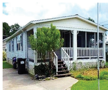
5363 McCLEARY LN CHINCOTEAGUE Own your own piece of the island in Misty Meadows! One-level living in this well-kept area! LOTS of new updates, including flooring for the entire length of house. Outbuildings for all your beach toys AND it's being sold completely furnished! WOW! Just $169,000
