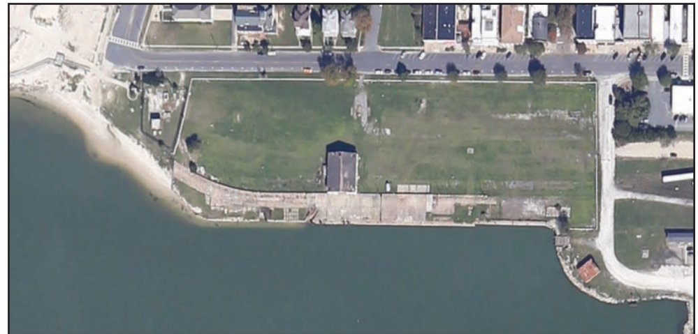
An aerial photo of the proposed development site on Mason Avenue.
