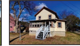
Chincoteague - Classic 2BR/1BA home with new plumbing and septic installed. Work in progress, but priced to sell! MLS# 46774 $115,000
