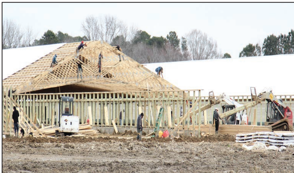
Chicken houses under construction at Chancetown.
