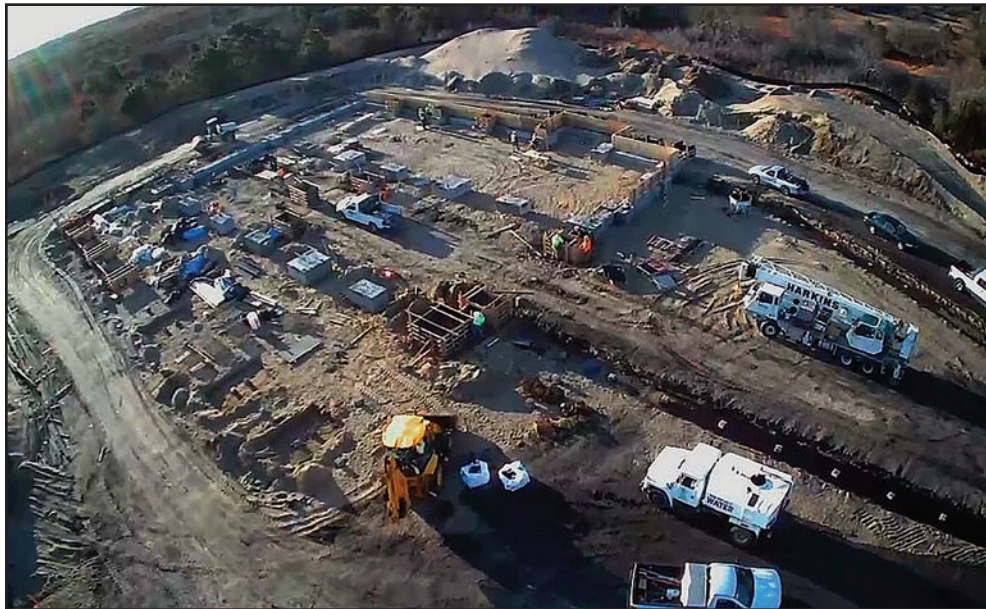
Aerial photograph of site preparation for new NASA payload processing center.
