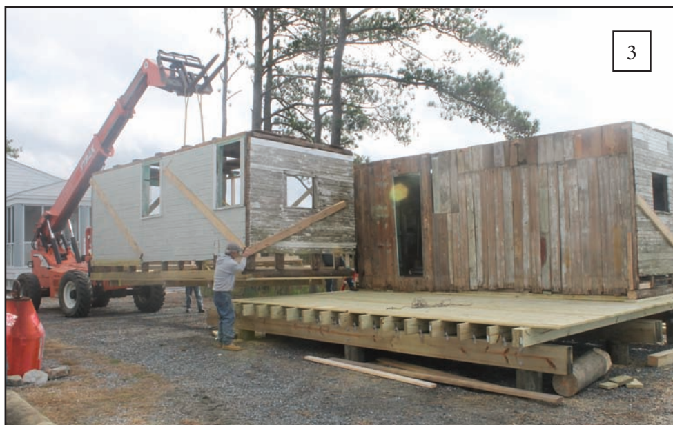
1. Half of workshop on a flatbed trailer, arriving at the museum. 2. Half of workshop in place on new deck foundation. 3. Moving the second half of the workshop into place on the new deck foundation. 4. Both halves of the workshop side-by-side on the new foundation.
