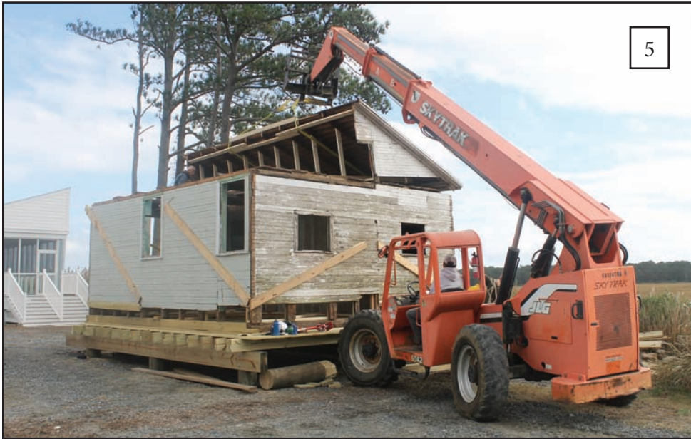
5. Lifting the roof into place.
