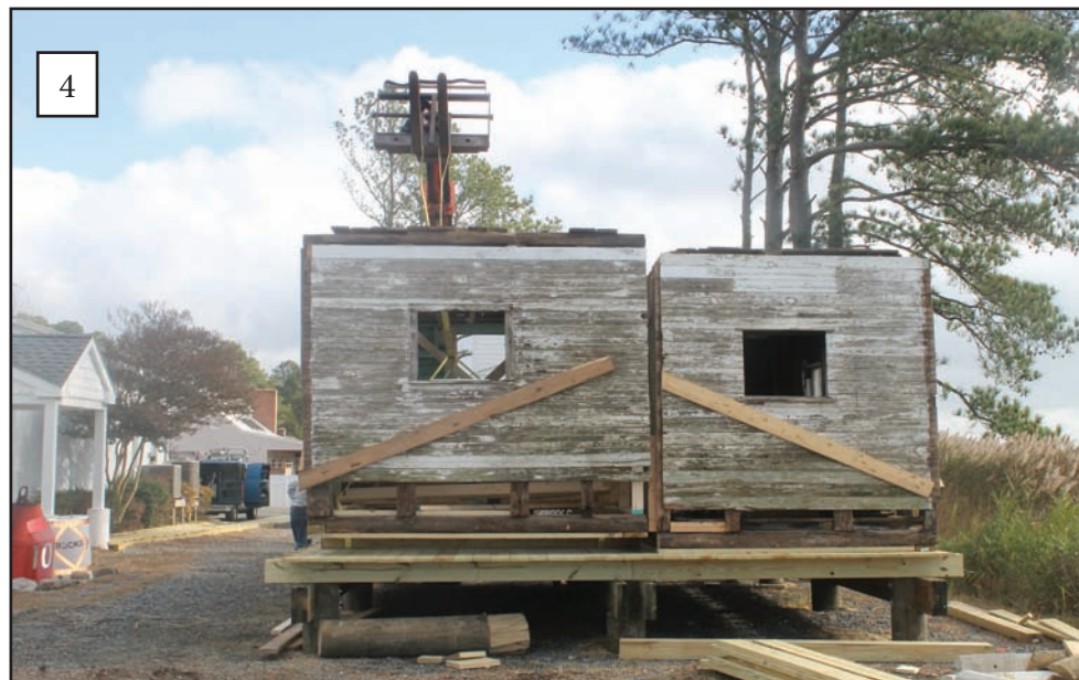
1. Half of workshop on a flatbed trailer, arriving at the museum. 2. Half of workshop in place on new deck foundation. 3. Moving the second half of the workshop into place on the new deck foundation. 4. Both halves of the workshop side-by-side on the new foundation.
