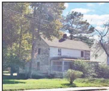
EXMORE, VA MLS 44532 $59,000- NEW LISTING- This home is a fixer upper on a .19 acre lot in the Village of Exmore. 2 bedrooms & 1 full bath. Has had roof replaced.
