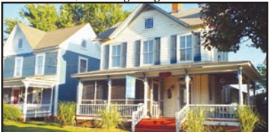
CAPE CHARLES: Loads of charm & comfort found in this 3BR/2BA Beach home. Enclosed front porch, foyer w/built-in bookcase, formal dining room, kitchen w/separate work areas, back staircase & open wrap-around porch. MLS#43479 $245,000 Kathy Weiner 757-646-3199
