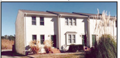
CHINCOTEAGUE: Immaculate 2BR/2.5BA end unit Mulberry Square Townhouse. Recent upgrades include HVAC, roof, fencing & septic. Turn-key ready & offers plenty of parking for your cars and boat. MLS#42227 $161,000 Gladys Baczek 757-894-0098
