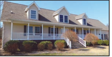
NANDUA BAY: Pride of ownership shows in this 3BR/3BA Cape Cod. Kitchen w/tile floor, custom counters & oak cabinets. 1st floor MBR, 2nd floor great room, rear deck & 2-car attached garage. MLS#42999 $289,000 Dave Griffith 757-647-2649/Randy Carlson 757-678-6395
